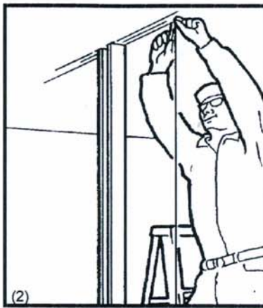
(2) Use a plumb bob or laser to transfer center line onto ceiling.
